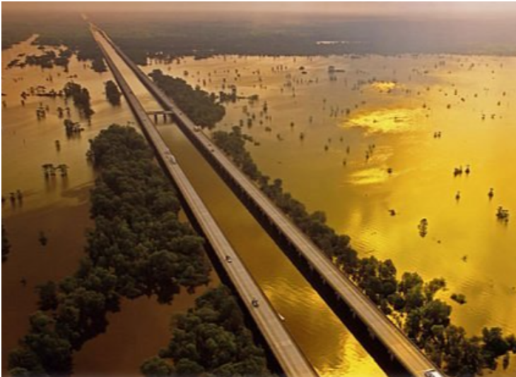
Figure: Atchafalaya Basin Bridge
